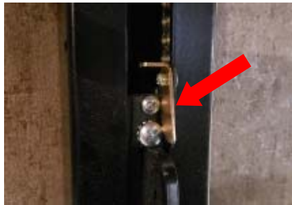
Figure 2. The picture above shows the locking tab in the 'Locking' position.
