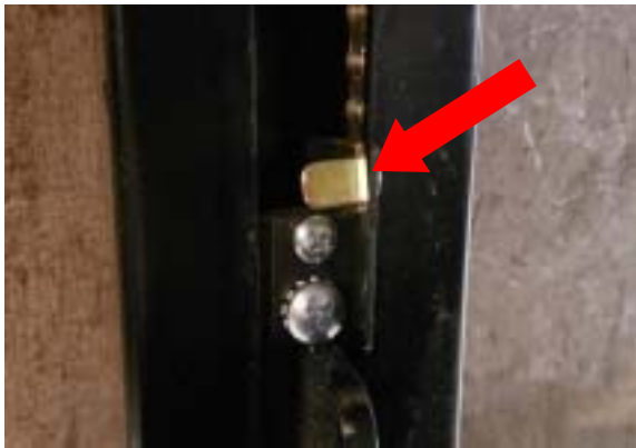
Figure 1. The picture above shows the locking tab in the 'Release' position.
